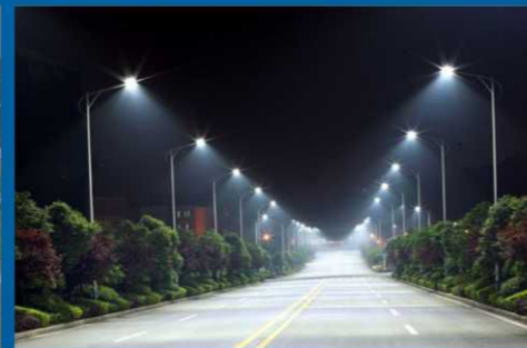
LED Street Lights
